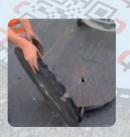
Manually remove the pavement around the manhole cover and recycle it.
